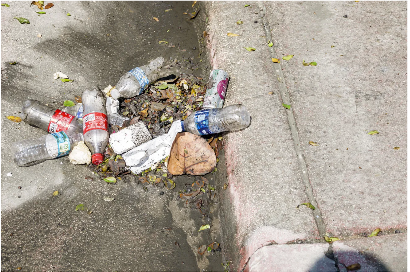
A drain in Miami Beach, Florida, clogged with plastic waste. | Jeffrey Greenberg/Universal Images Group via Getty Images
