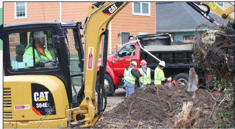
Removal of unsafe lead begins in contaminated Atlanta neighborhood
