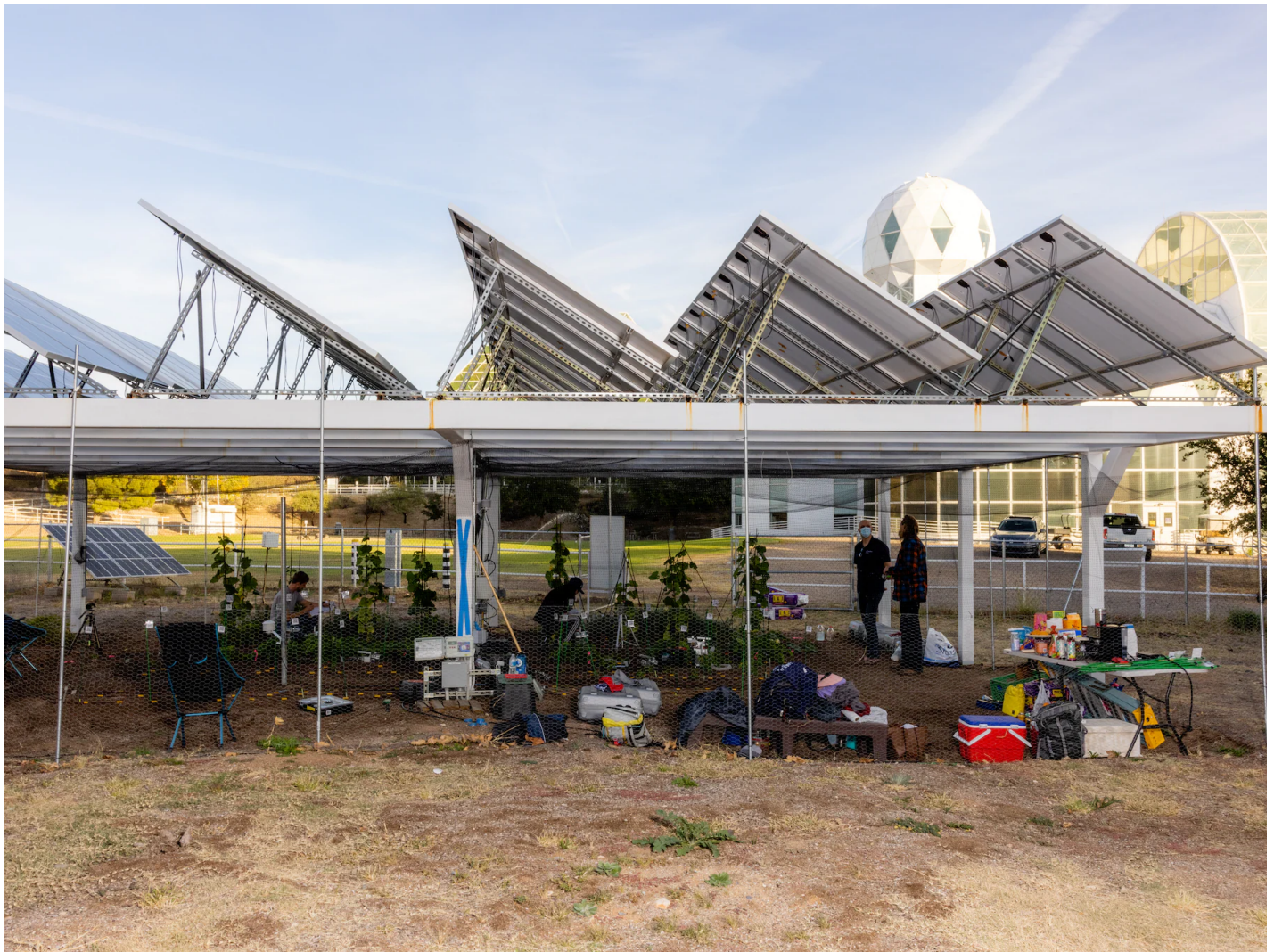
Crops are grown under a solar canopy that is key to an agrivoltaic project at Biosphere 2 in southern Arizona.
